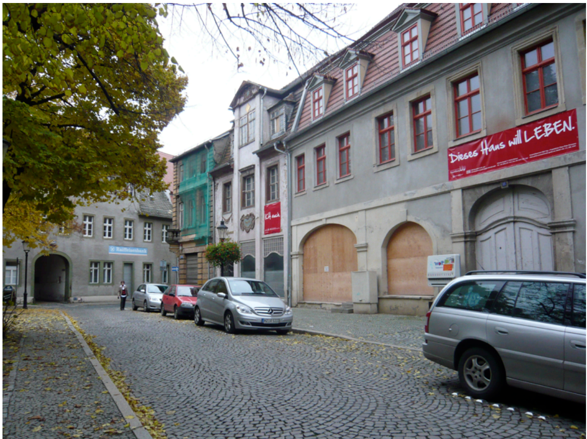
Fig. 3.11 The rest of the street also wants to live
