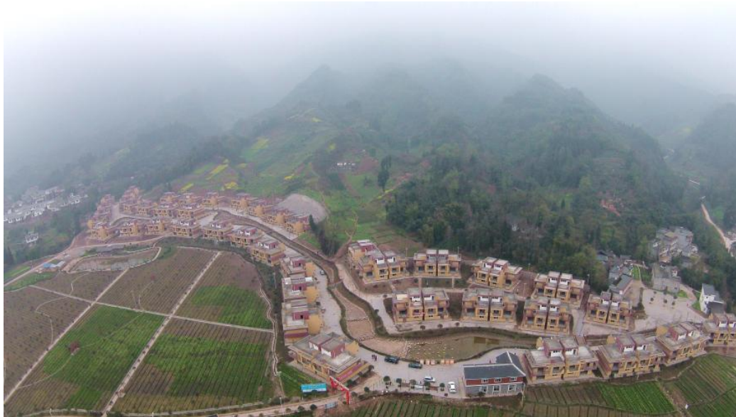
Figure 1: Rebuilt housing estate in S township
