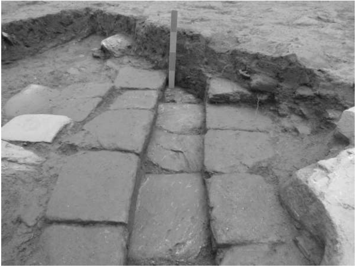
Figure 19: Detail of stone lined drain looking west.
