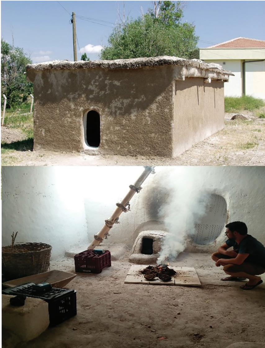
Figure 4. A reconstructed building at Çatalhöyük. Photograph by Lisa-Marie Shillito.
