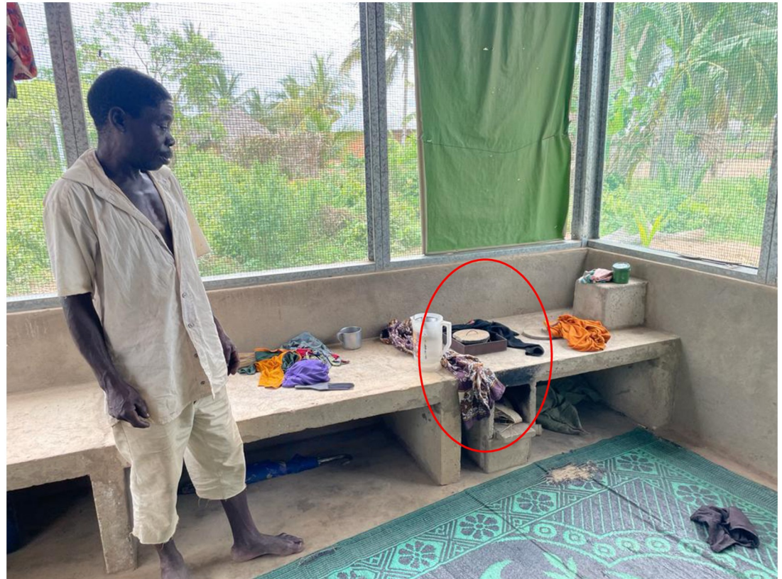
Fig 3. A Star home resident showed his stove and a shield (marked by a red ring) on the shade net. The issue of water ingress on the ground floor was also raised by residents. This was despite occasional holes in the shade nets being fixed by the Star Homes team. Sometimes, the stove fire was extinguished by the rainwater coming into the kitchen.
