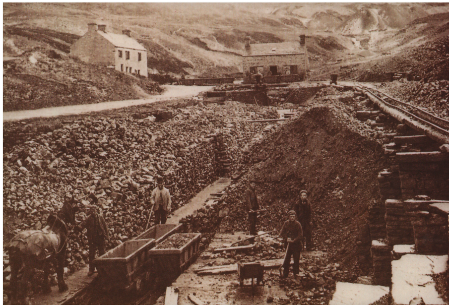
Fig. 4. Historical photograph (c. late 19th century) of Smallcleugh Mine, Nenthead, showing miners loading ore from the bouse teams (storage bins) ahead of ore dressing work at Rampgill Mill. The extensive disturbance and mine waste tips throughout the upper Nent catchment can be seen in the background, with the River Nent itself channelised immediately alongside the track to the left of the photograph. Processing waste from this period of mining was often deposited close to the river or even discharged directly into the channel. Image © The Simon Danby Collection, 2021.
