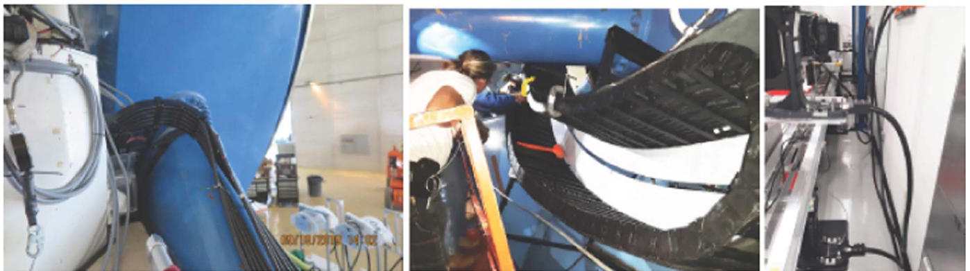
Figure 42. The fiber cables are stored in articulated cable carriers (e-chains) in order to guide them around the axis of the telescope. The middle panel shows the polar axis being inspected in order to ensure that it moves smoothly and without obstructions. The panel on the left shows the cables as they route over the telescope truss before penetrating the wall of the spectrograph shack. The panel on the right shows the cables in the spectrograph room attached to their science slits. This process is shown schematically in Figure 13.
