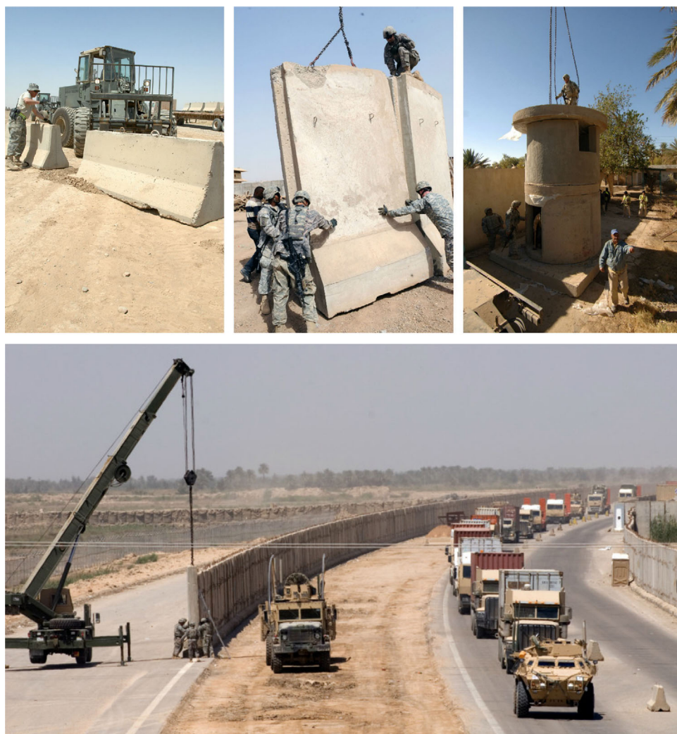
Figure 1: Top—Images of emplacing [i] Jersey walls (far left), [ii] Alaska blast walls (centre), and [iii] guard towers used at checkpoints (far right) in Iraq 2008. Image credit: Senior Airman Eunique Stevens, US Air Force; Staff Sgt. James Selesnick, US Army (source: Spencer 2016). Bottom—the US military's tactic of lining every major road with T-walls. Image credit: Spc. Kiyoshi Freeman, US Army (source: Spencer 2016).
