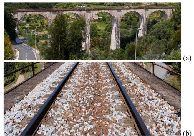
Fig. 1. Quebradas viaduct: (a) global view of the bridge and (b) detail of the railway track.
