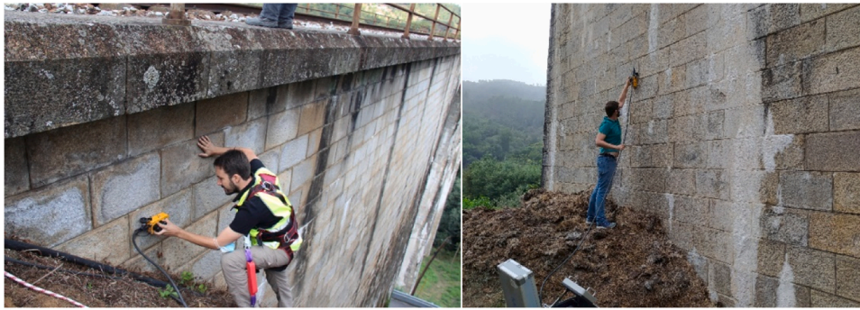
Fig. 18. GPR tests at two different locations of the bridge.
