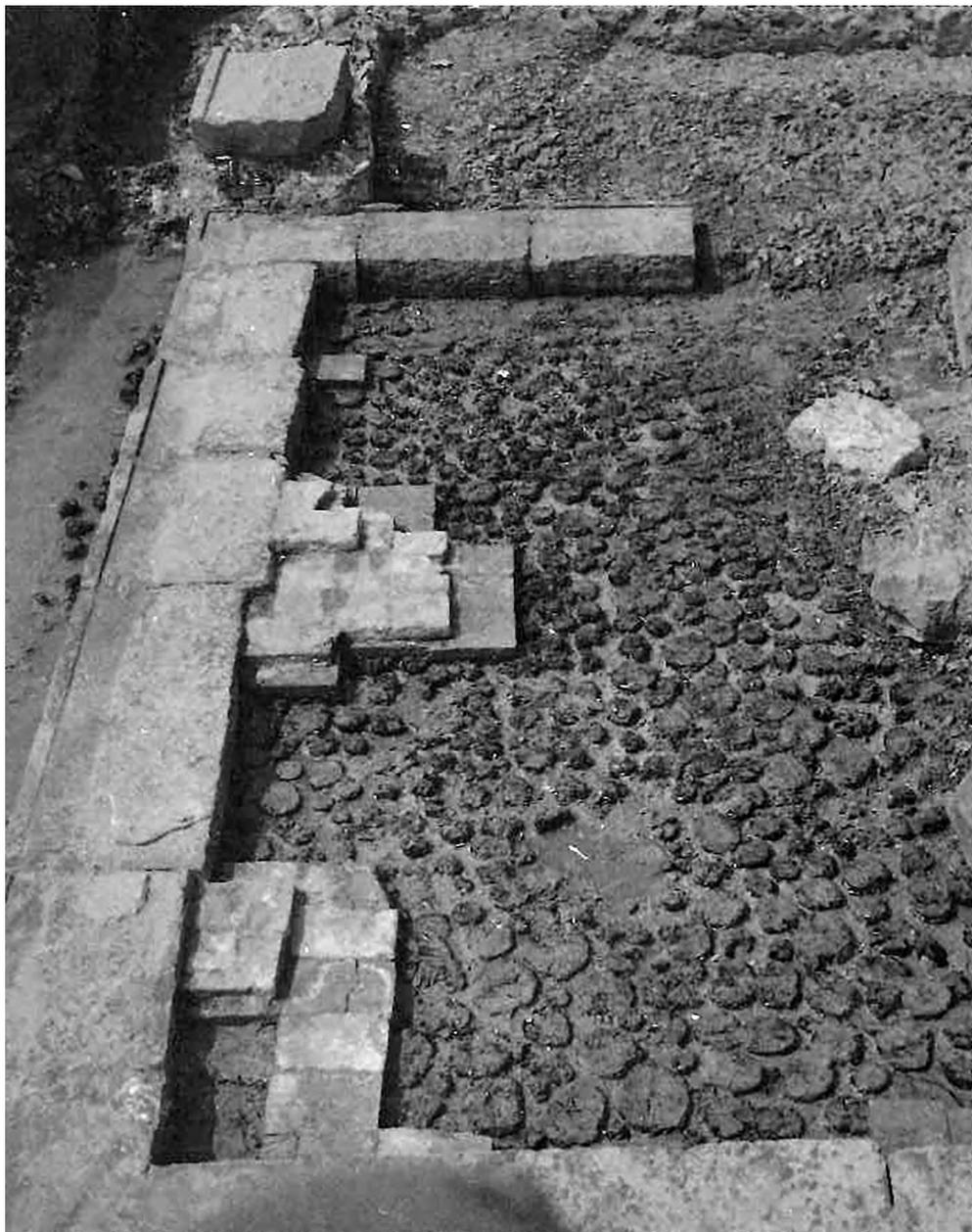
Fig. 5.—Preparation of the soil: piles underneath a huge monument along the north ditch of Annia (from Scarfi, 1985).
