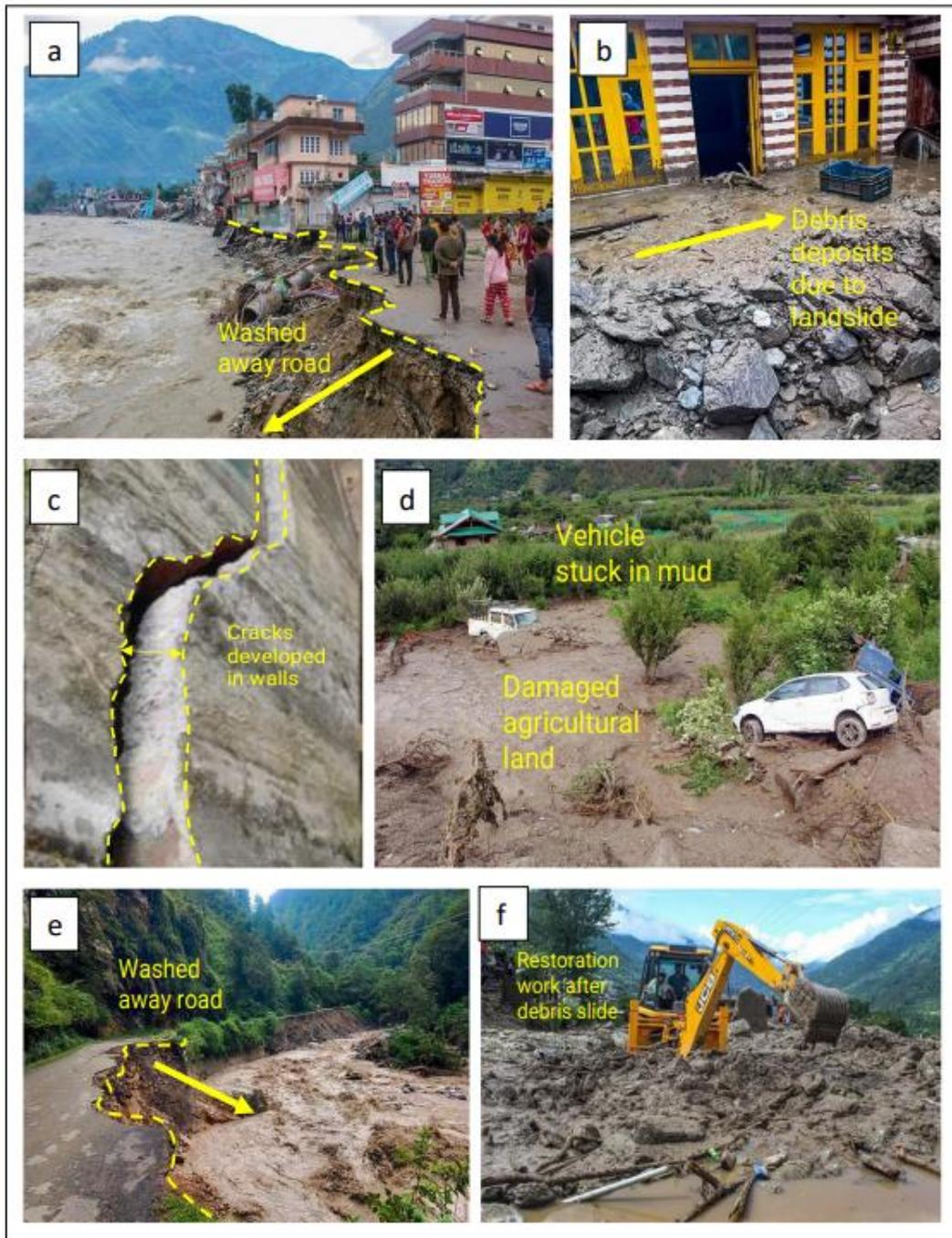
Fig. 5 Damages in the Kullu district. **a** Washed away road section (India Today 2023b), **b** Debris deposition in front of houses (Outlook 2023), **c** Cracks in houses (ETV Bharat 2023), **d** Damaged agricultural land and vehicles due to mud slide (The Tribune 2023e), **e** Washed away road section (The New Indian Express 2023), **f** Restoration work after a debris slide (Outlook 2023)
