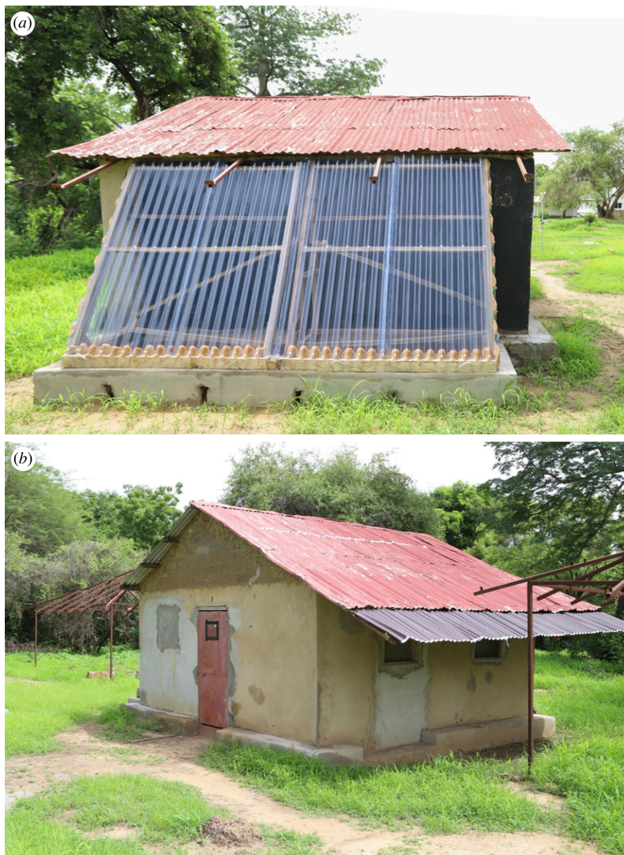
Figure 3. Experimental house with solar chimney on southeast facing wall (a) and extended roof on northwest elevation (b).
