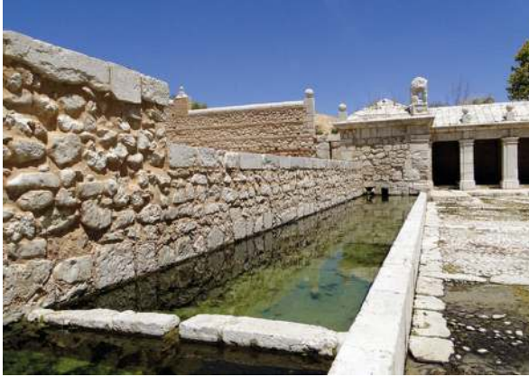
Fig. 10 The 'Great Fountain' at Ocaña, Toledo, constructed in 1573–1578.
