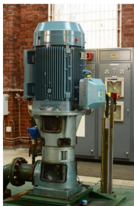
Fig 1. 110kW SynRM at Somerford Pumping Station [2]
