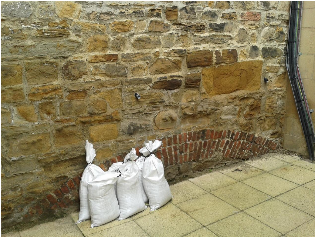
Figure 4: Brick relieving arch at the rear of the western stable block of likely late 17 th or early 18 th century date.
