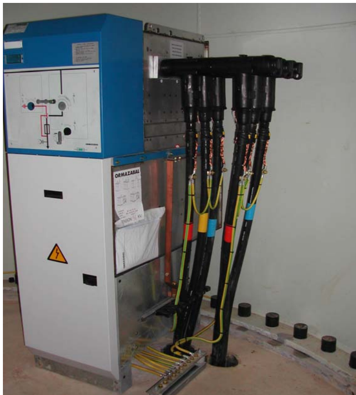
Figure 4: Physical arrangement of a separable “T” arrangement
