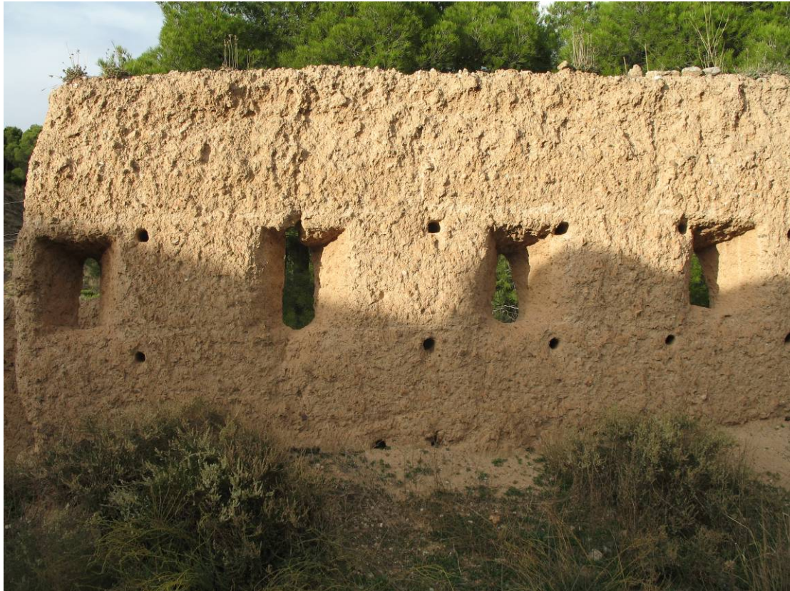
Figure 9: Rammed earth wall, Daroca. Constructed 1837, windows are rifle ports. (Photograph Jaquin 2007)
