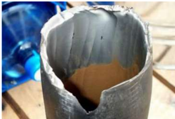
Figure 3. Pipeline after failure due to stress cracking (reproduced with permission from ref. 27).
