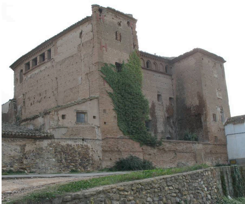
Fig. 1. The preceptory at Ambel, north-east elevation. The gallery of arches between the towers is typical of 16th century architecture in this region. The first phase precinct wall reaches the base of ivy and stands 3m high.
