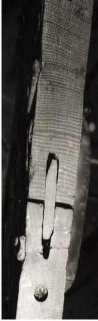
Figure 3: Cross Section Through Plank 2 (Q8795), West Leaf of the South (Monk's) Door: Photograph by Trevor Woods, Department of Archaeology, University of Durham Note the free tenons between the mortised planks and the circular holes resulting from the removal of the samples for radiocarbon dating.
