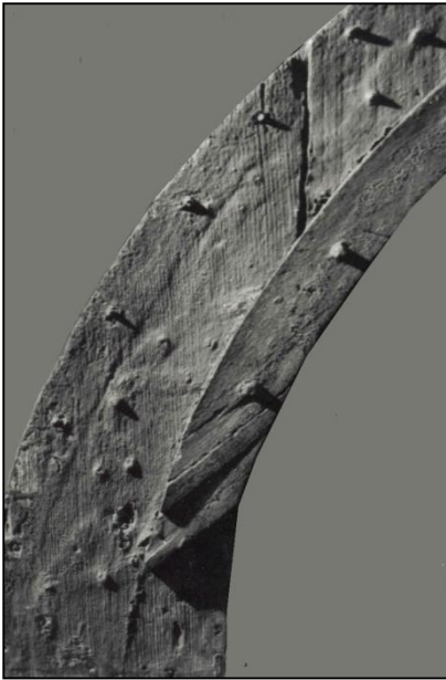
Figure 5: Upper front face of the East Leaf of the North Door during restoration. Photographed in raking light by Trevor Woods, Department of Archaeology, University of Durham. Note the corroded nailshanks and raised ridges of the original strapwork
