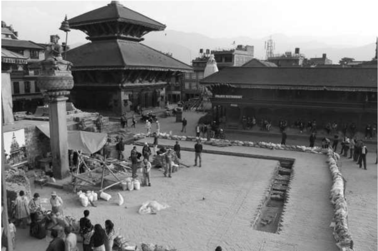
Figure 5: General view of Trench 1, looking south over the Durbar Square.
