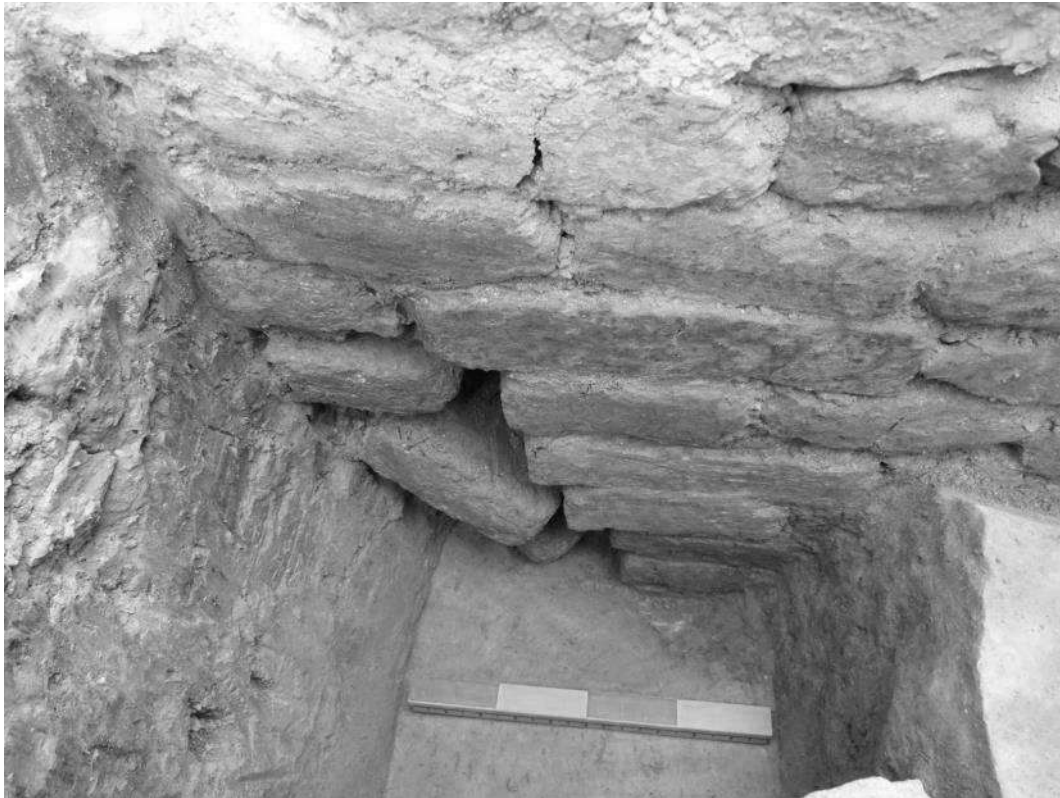
Figure 10: Shear crack of wall within Trench 1 indicating possible earthquake damage.
