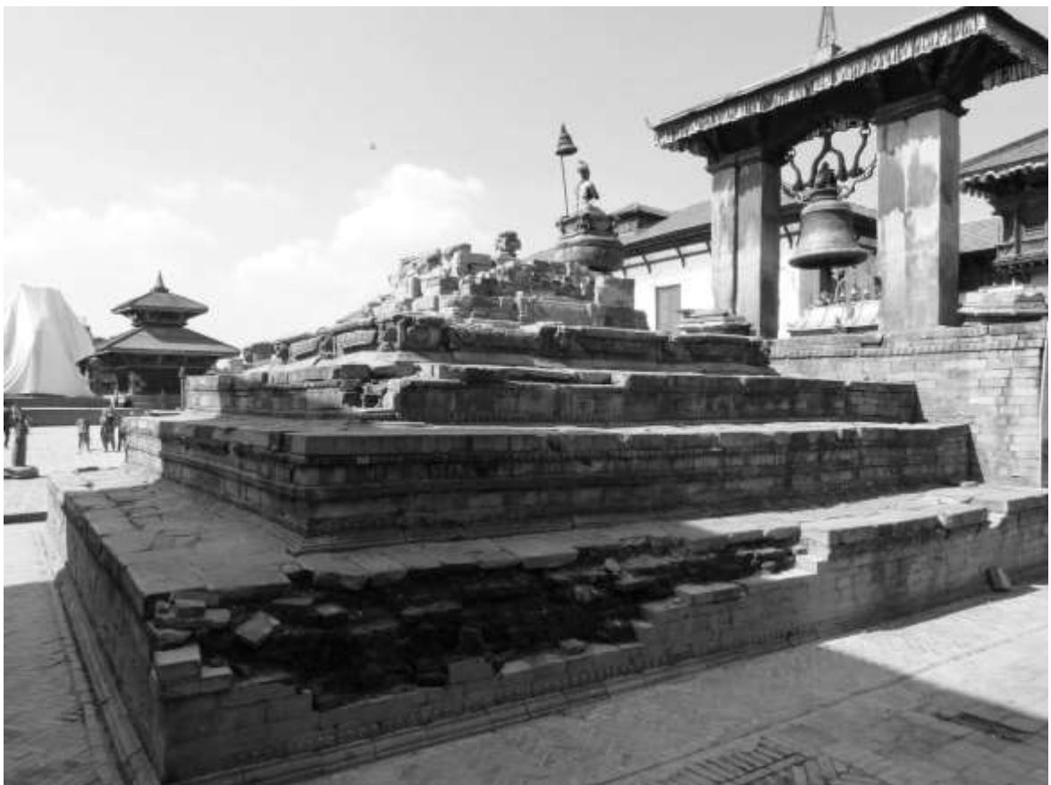
Figure 4: The collapsed Vatsala Temple on surviving plinth.
