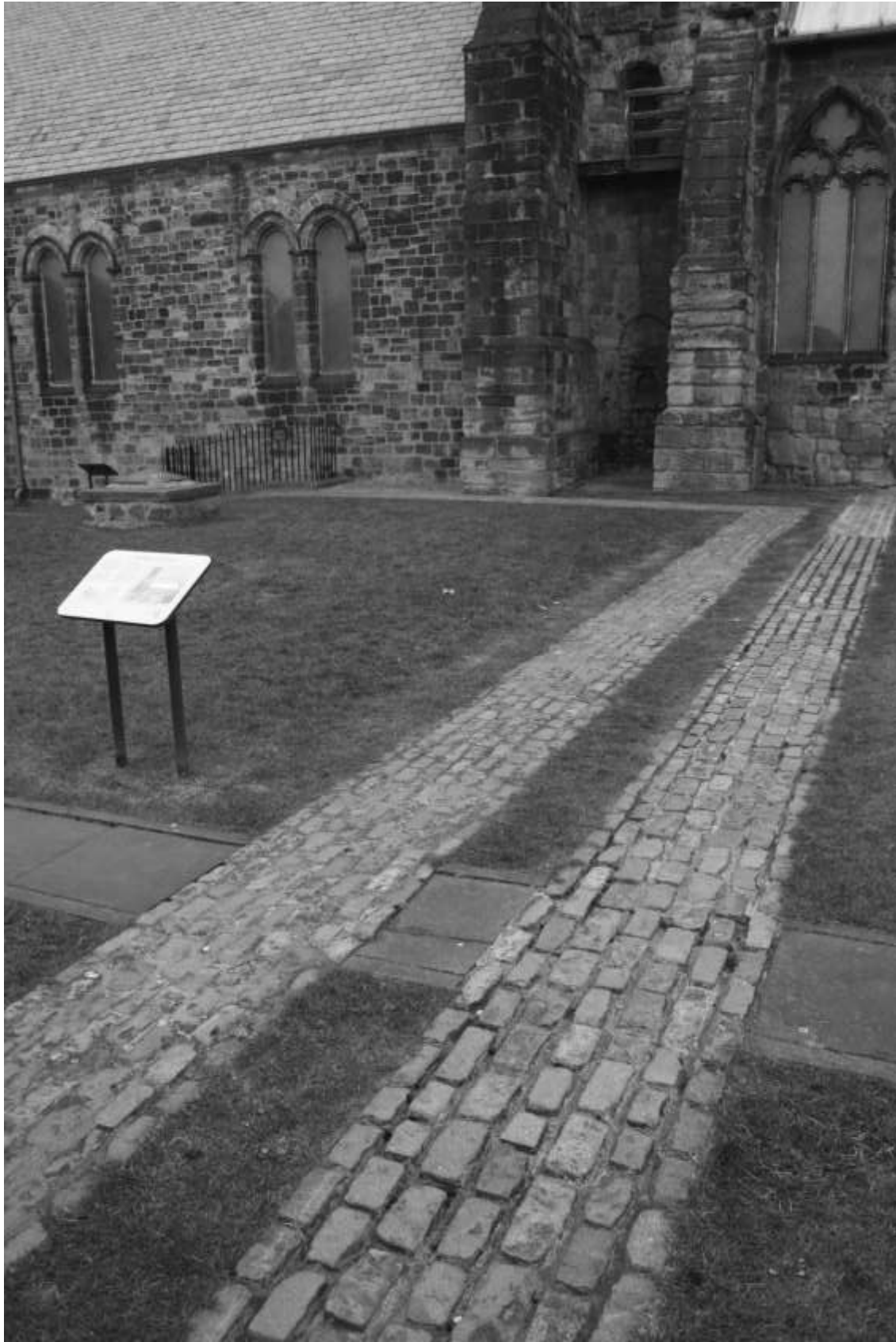
Figure 26: Different phases of subsurface wall alignments represented through differing brick patterns at the site of Jarrow, United Kingdom.
