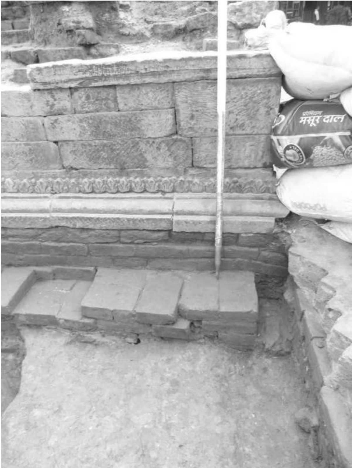
Figure 13: Later brick courses overlying earlier footprint of the Vatsala Temple at the south-west corner.
