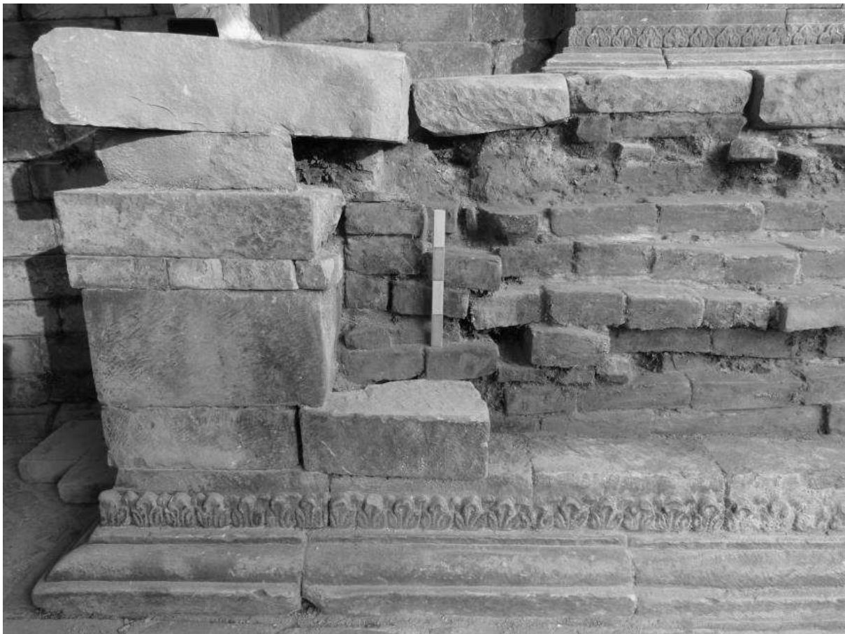
Figure 19: Differing phases of construction and bonding of brick and stone block masonry in Trench 1B.
