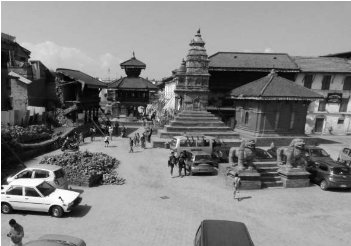
Figure 2: Earthquake damage in Bhaktapur's Durbar Square.
