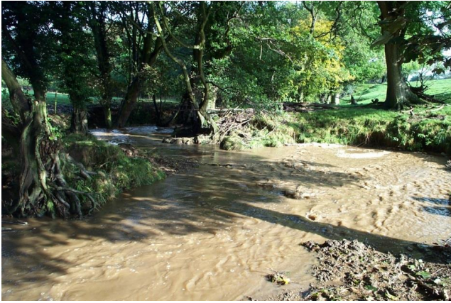
Figure 4. View looking downstream of the channel diversion during the construction phase. Photograph taken on day of diversion works; 10 October 2007.
