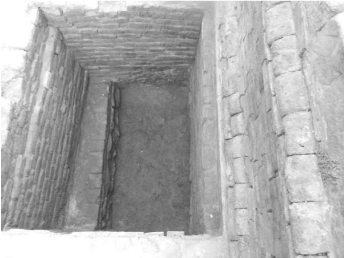
Figure 20: Stone cobble foundations visible in trench cleaned by the team that was left open by KVPT on the western side of the Char Narayan Temple, looking north.
