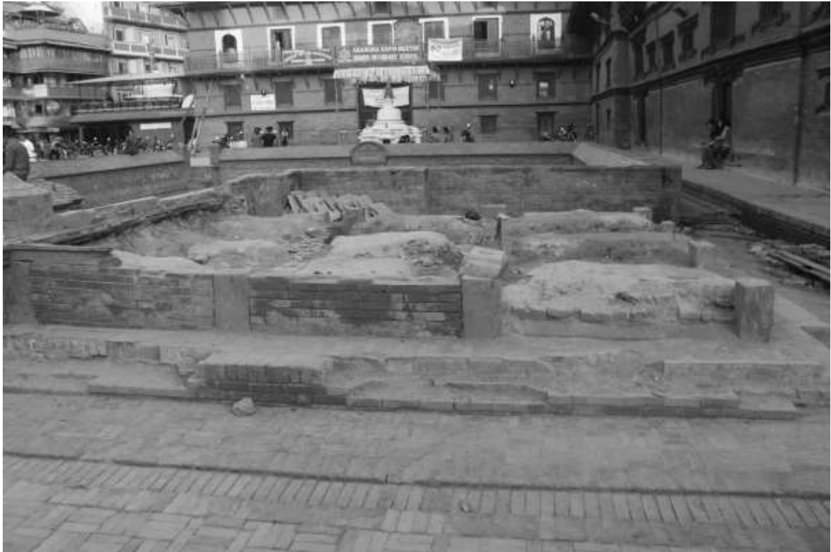
Figure 2: The collapsed Mani Mandapa, looking east.
