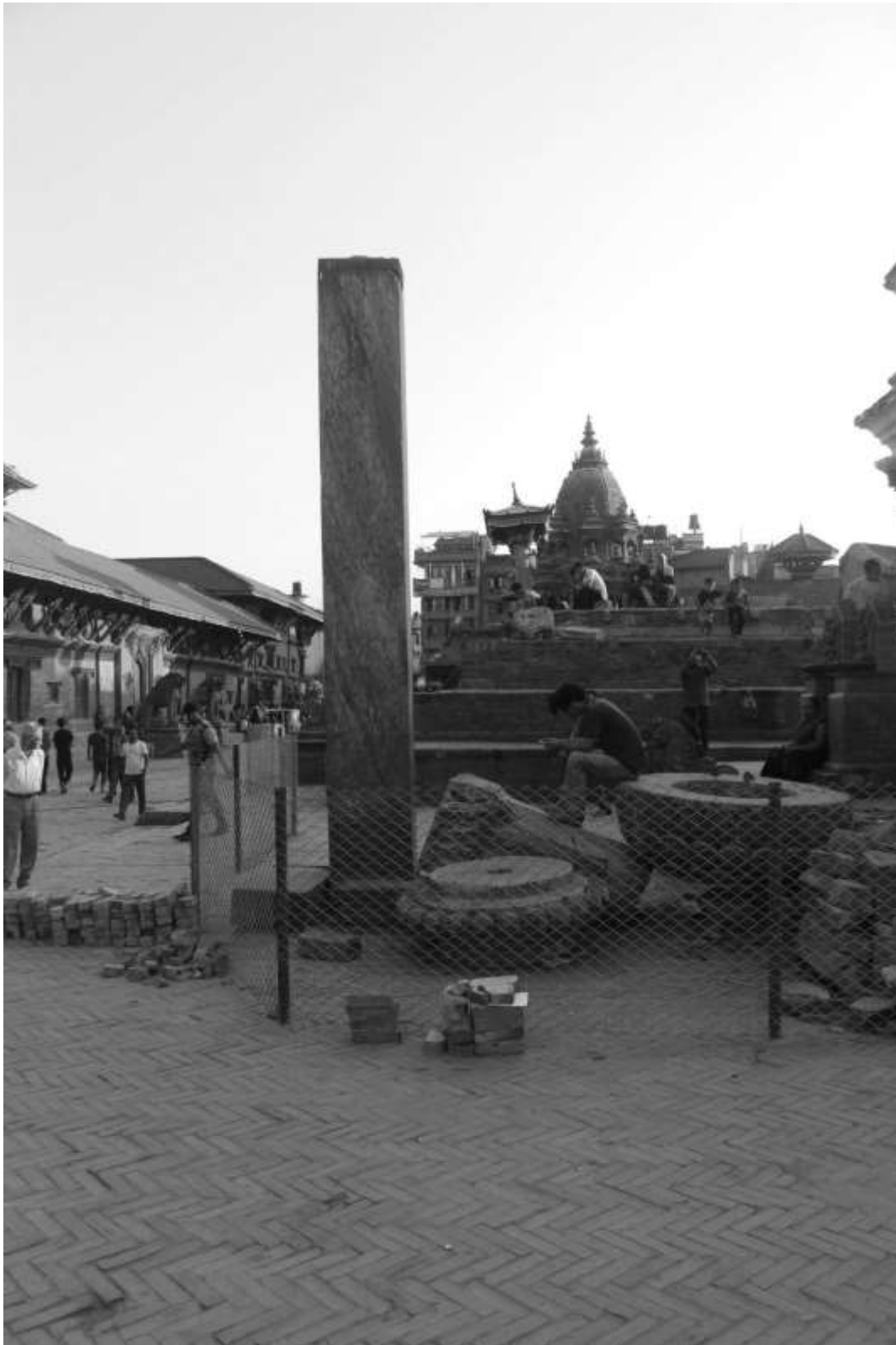
Figure 1: Damage in Patan's Durbar Square, including the damaged pillar of the statue of King Siddhi Narasingh Malla, and the collapsed Harishankar Temple, looking south.
