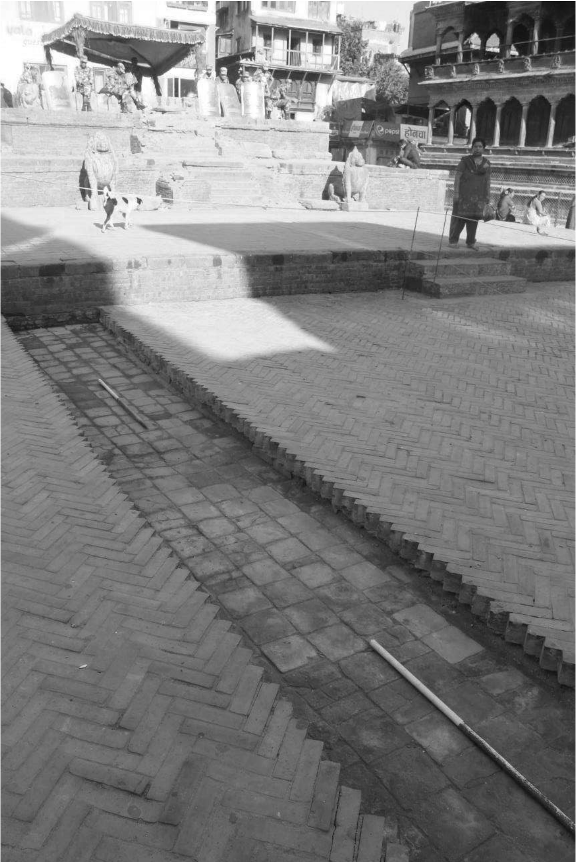
Figure 4: Tiled paving surface below the current paved Durbar Square, in Trench 1A.
