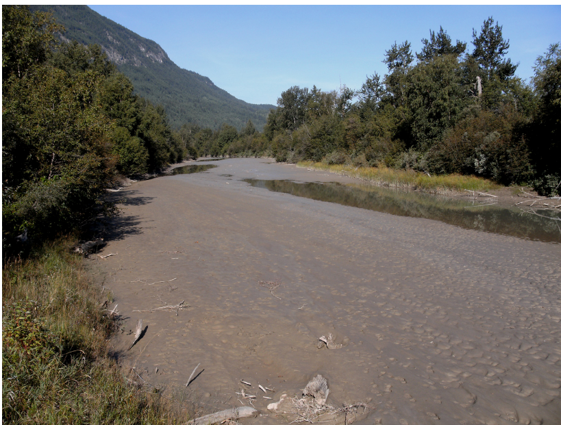
Fig. 7. Channel 3 in the Harrogate cross-section, which has almost completely filled with sand. Channel width is ca 40 m.
