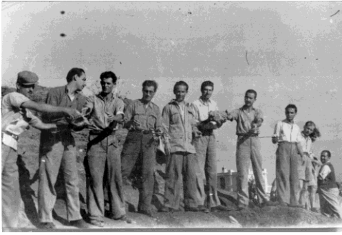
Figure 1: Group of exiles working on the construction of a road in Ikaria, 1947. (Author: Kassimatis, Archive of Christos Malachias)
