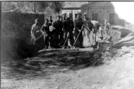
Figure 2: Group of exiles working on the construction of a road in Ikaria, 1947. (Archive of Christos Malachias)
