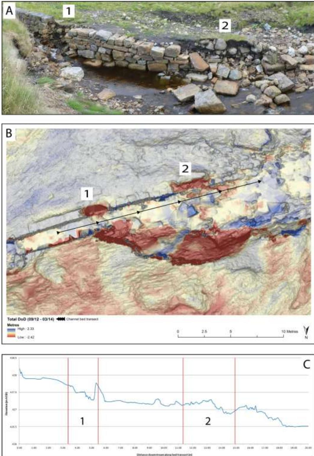
Figure 6 – Collapsed sections of the drystone retaining wall adjacent to the upper dressing floor at Whitesike Mine as seen in a field photograph from September 2013 (A) and the overall 18 month DEM of Difference (B). The relationship between the collapsed sections and the dGPS measured bed elevation profile of Garrigill Burn is shown in the associated line graph (C). Numbers 1 and 2 represent the locations of corresponding collapsed sections on each of the figure panels.
