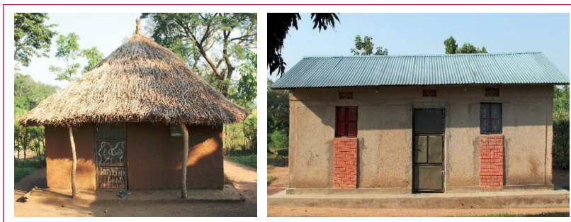
Figure 1: Traditional (left) and modern (right) houses in rural Uganda Traditional housing is typically characterised by thatched roofs, mud walls, and open eaves, whereas modern housing is built with metal roofs, concrete or brick walls, and closed eaves.
