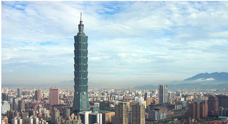
Fig. 12. Top: The Taipei 101 building, Taiwan ( http://inhabitat.com/taipei-101-worlds-tallest-green-building/green-taipei-101-1 ). Bottom: Earthquake history for a 16-year period spanning the construction of the building. (From Lin (2005).)
