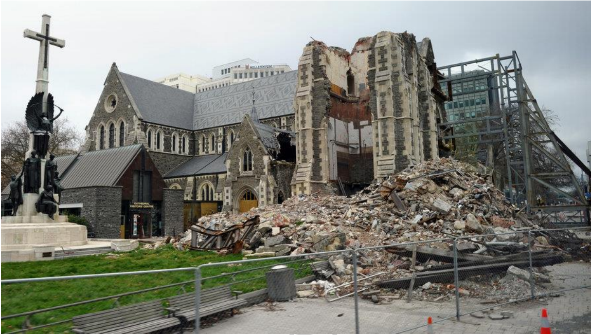
Figure 114: Damage done to the cathedral in Canterbury, New Zealand, by the 2010 M 7.1 earthquake 22 .
