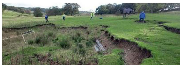
Case Study 2: Erosion Exposing High Pressure Gas Main, Brancepeth Beck
