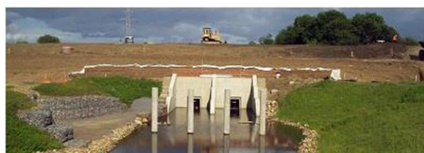
Case Study 3: Sedimentation of Culvert Under Dam, River Gaunless
