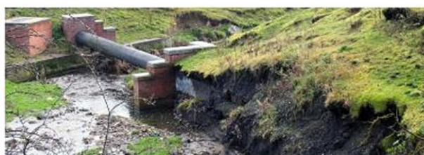
Case Study 4: Erosion Undermining Mains Water Pipe, Crook Beck
