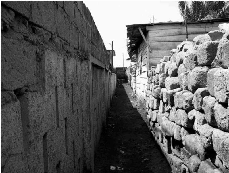
Figure 4. Passageway showing concrete, stone, and timber walls.
