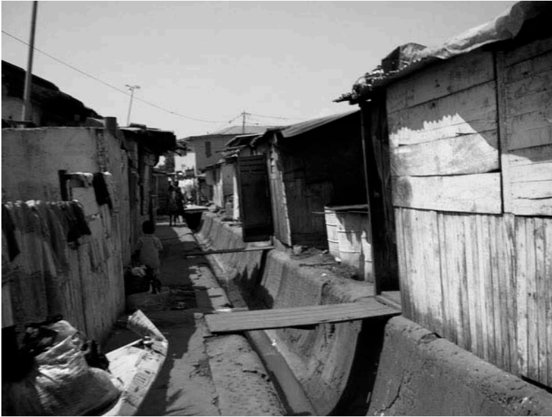
Figure 3. Timber-constructed walkway over sewerage.
