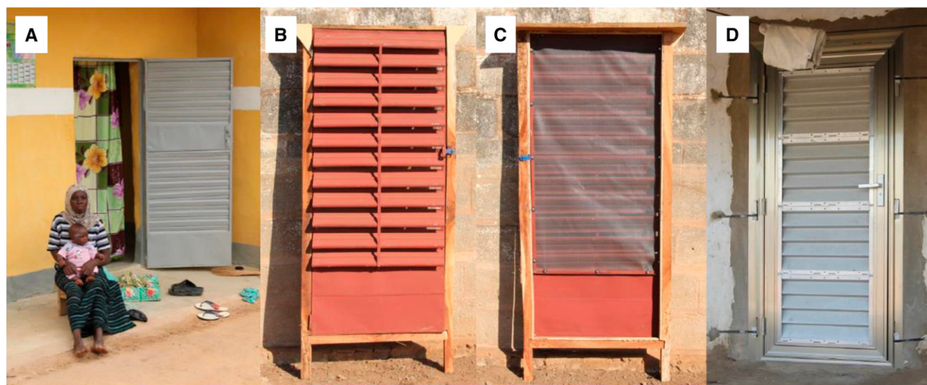
FIGURE 1. Evolution of the louvered door. (A) Typical unscreened Francophone door from West Africa; (B) RooPfs door external view; (C) RooPfs door internal view, showing screening and (D), the concertinaed screened door, D1. This figure appears in color at www.ajtmh.org .
