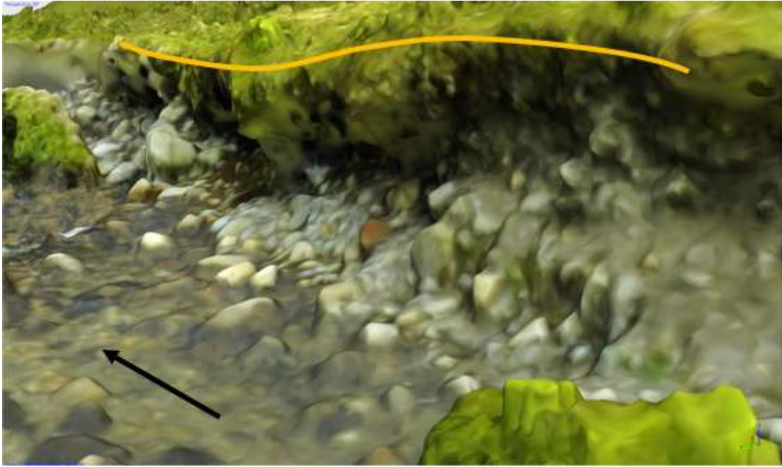
Figure 10: PAP_HQ model close-up illustrating a capacity to capture overhanging bank features. See Figures 2 and 3 for exact feature location. Orange line represents a 6.5 m section along the right riverbank. Arrow indicates flow direction.
