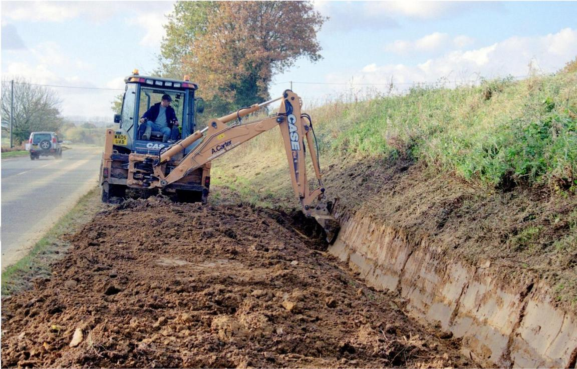
Figure 11. Ditch being dug to protect A272 road from muddy flooding, 01/11/2008, Slade Lane, Rogate, West Sussex
