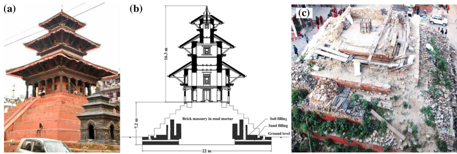
Fig. 3 Jaisidewal temple: a schematic representation of the temple (Image: ICOMOS, Nepal) and b photograph before 25 April 2015 (Department of Archaeology, Nepal), c photograph after 25 April 2015 (Reconnaissance survey)
