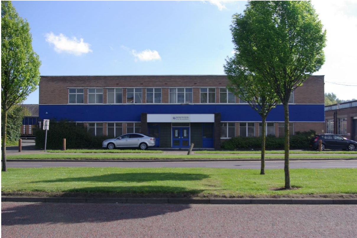
Fig 16 The west (front) elevation of L50. The entrance was rebuilt in the early 1970s and prior to this the first-floor was extended to the full length of the frontage. This is not apparent in the brickwork as the colour has been very carefully matched, though there are joints apparent in the concrete lintel above the windows.
