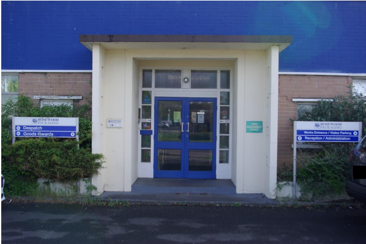
Fig 13 photograph of L92 entrance, apart from the door itself this is the entrance built in 1939. Note the decorative canopy and planters to either side. The sides of the supports of the canopy are decorated with squares in relief.
