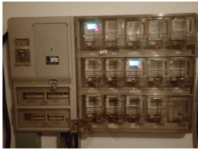
Figure 5: The combination of electricity meters in the basement.
