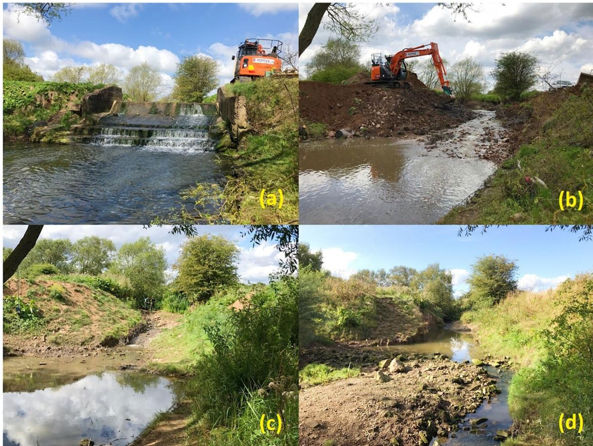
**FIGURE 2** Cluff Bridge weir on Claxton Beck before removal (a), immediately after removal on 30 April 2018 (b), five months after the weir removal (c), and 17 months after the weir removal (d). Photographs were taken under base flow conditions
