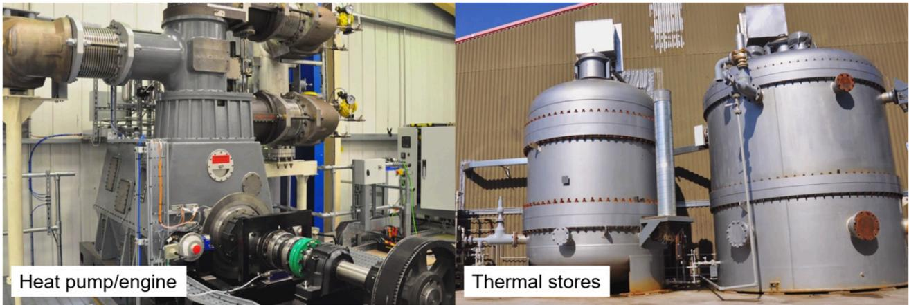
Fig. 1. 150 kW<sub>e</sub> PHEs demonstrator built at Hampshire, UK.
