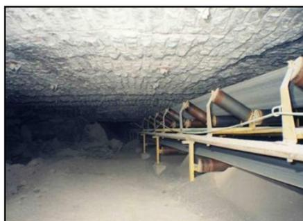
Figure 1: Ground squeezing observed at Boulby Mine [1].
