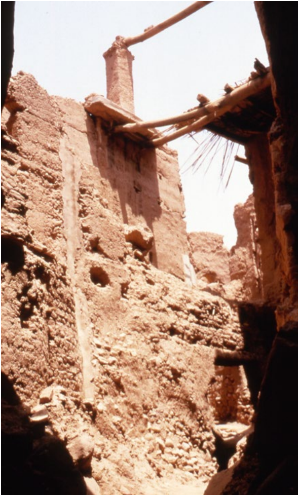
Figure 6.4. A deserted “ghost town” at Tinerhir in Southern Morocco (photos by Bernhard Epstein, left, and EWS, right). Collapsing mudbrick architecture not worth reusing is gradually resulting in the build-up of heaps of soil, the same well-known phenomenon we see in the barracks mounds in the forts on the Gorgān Wall.
