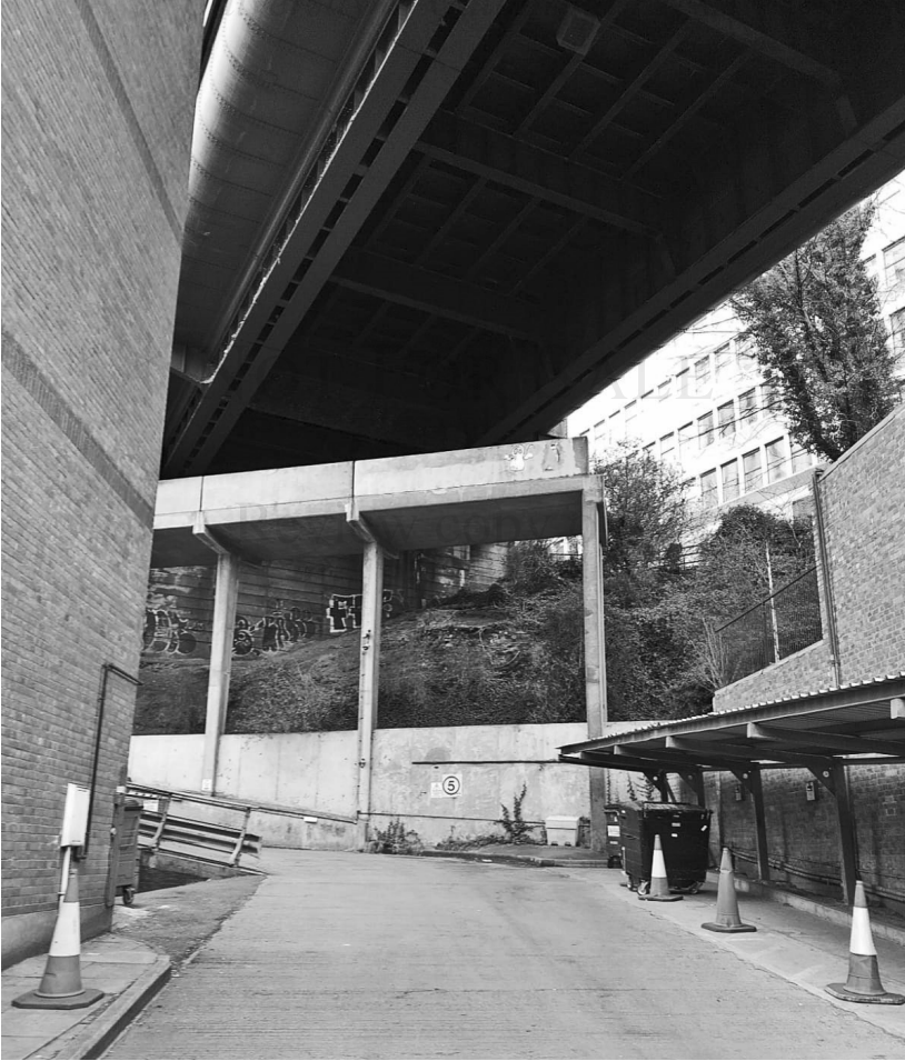
FIGURE 17. Unfinished walkway, Newcastle (PERMISSION?)
